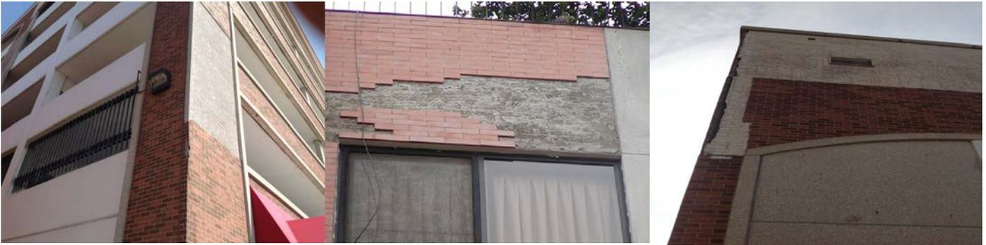
The absence of a systems manufacturer for consultation and field support resulted in an installation without a single control joint, and thus the buckling of walls. The entire building is being stripped and reinstalled.
