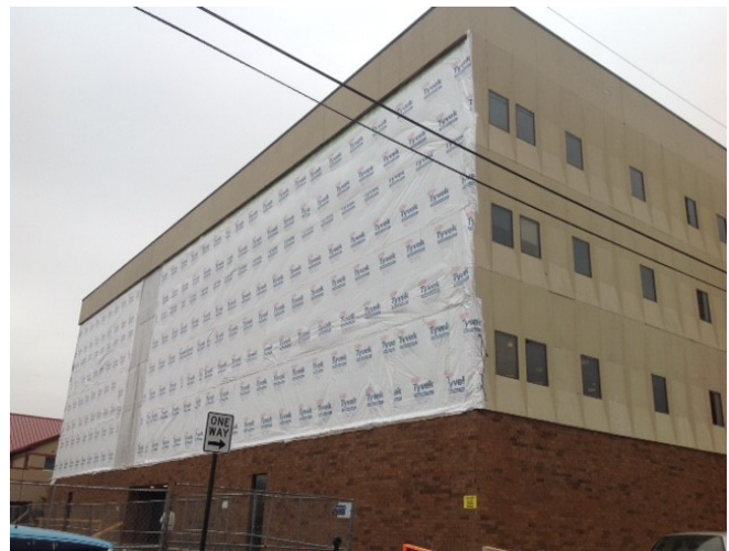
Removal of Precast
