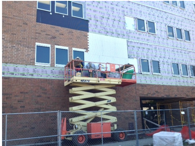
Installation in Progress
