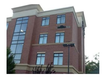
Insufficient fasteners (and non-galvanized fasteners) resulted a complete section of veneer falling below.
