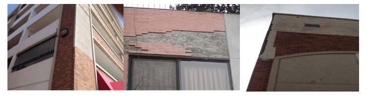
The absence of a systems manufacturer for consultation and field support resulted in an installation without a single control joint, and thus the buckling of walls. The entire building is being stripped and reinstalled.
