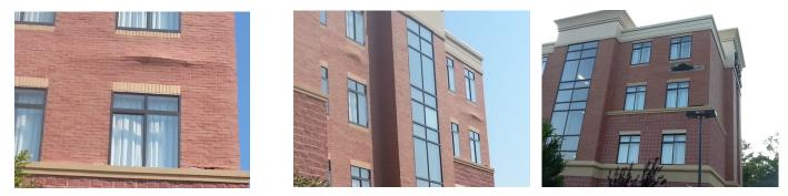
Three years ago, **TABS Wall Systems** received a call from a frantic hotel owner in Richmond, VA. The hotel had thin brick installed with a lath system. As visible in the photos, the walls were literally buckling.
