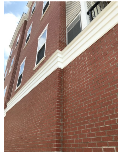
Corner Cracking at upper floors with wood framing; no cracking at 1st floor with steel framing
