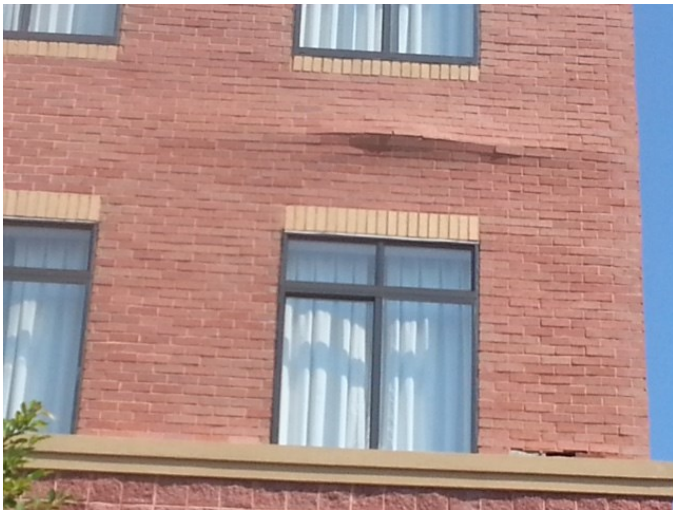
Floor Line Buckling Due to absence of control Joint
